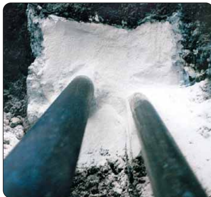
14 Year Old Installation
