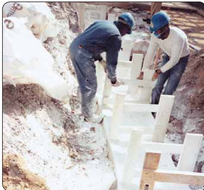
Removal of Temporary Spacers
