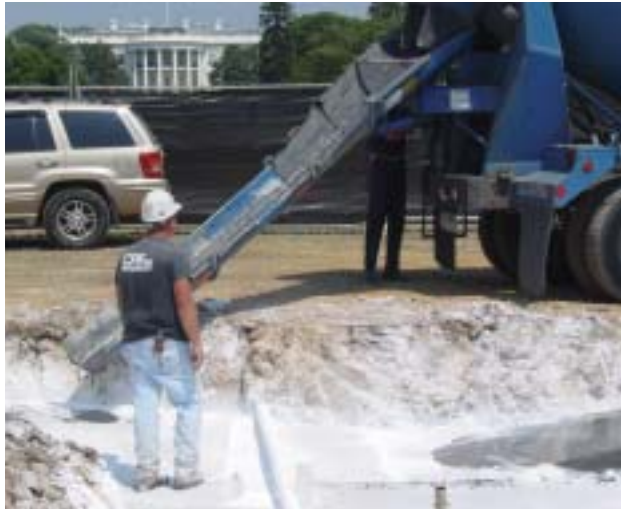
Flowable Fill cement being installed over DriTherm insulation.
